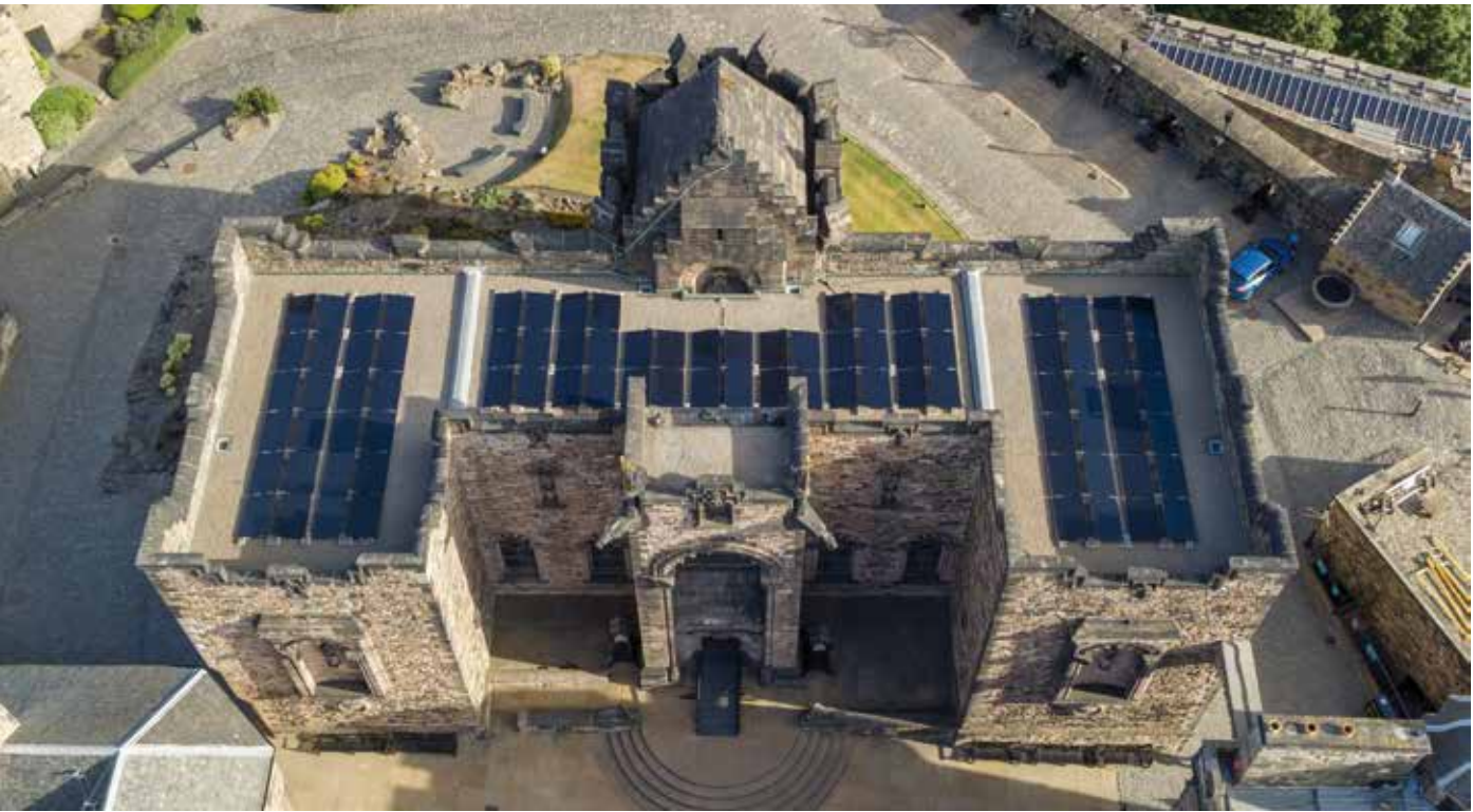
Paneles fotovoltaicos en el castillo de Edimburgo, Patrimonio Mundial. © Historic Environment Scotland (HES). National Collection of Aerial Photography (NCAP)
