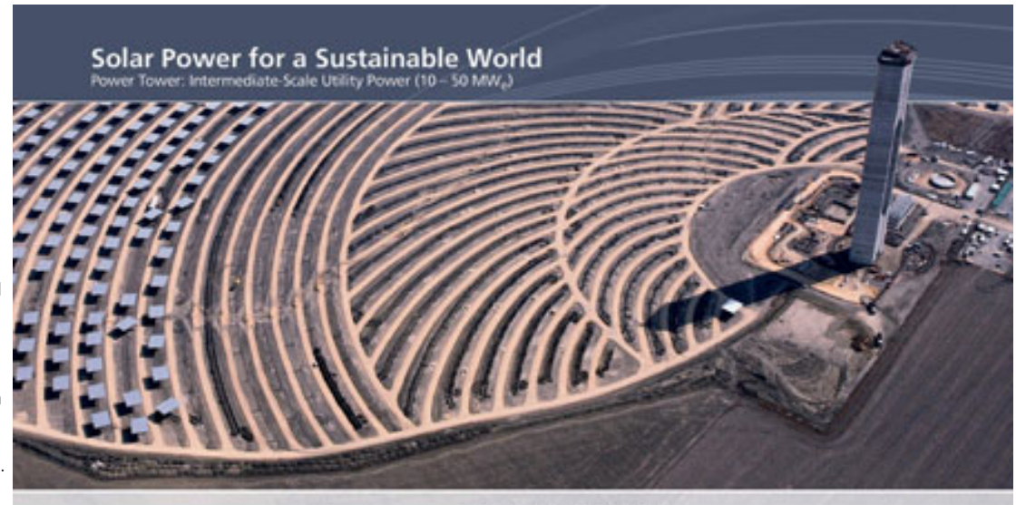
PS20 under construction in Spain
