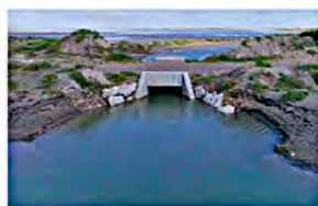
1 Rehabilitated water gate
