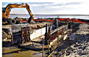
2 New water gate
