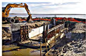
2 New water gate
