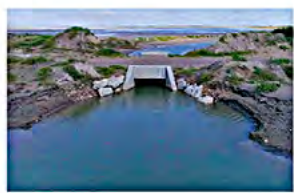
1 Rehabilitated water gate
